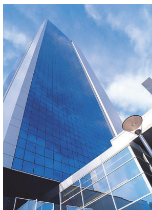
Figure 3. Polat Tower (retrieved on 20.02.2015, http://www.polattower.com/tr/sanalur )
