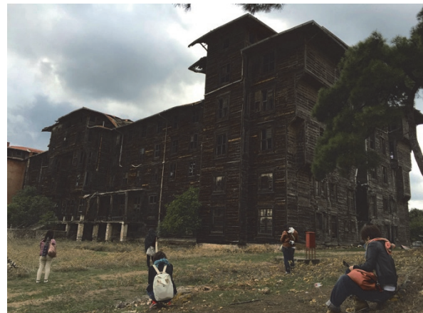
Making sketches of the Greek Orphanage carefully checking the ubiquitous elements of traditional Turkish house design
